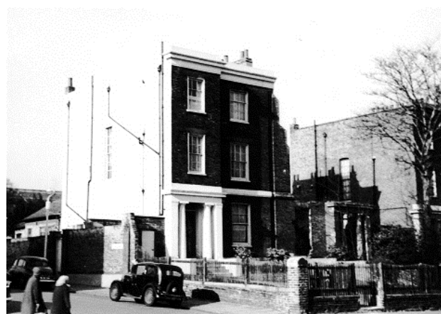
320 Brixton Rd, London SW9 – the SCRSS's home since 1969, photographed in 1947 (SCRSS Archive)
